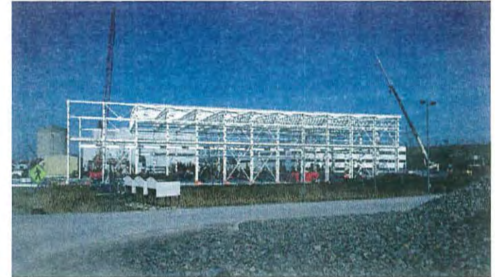
Erection of structural steel
