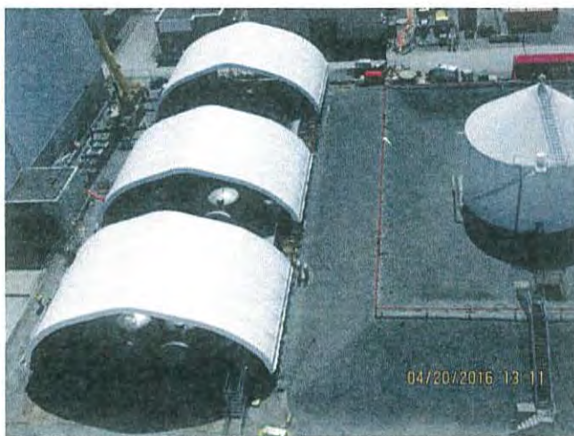
Installation of a temporary roof
