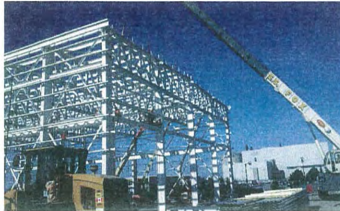
Erection of structural steel
